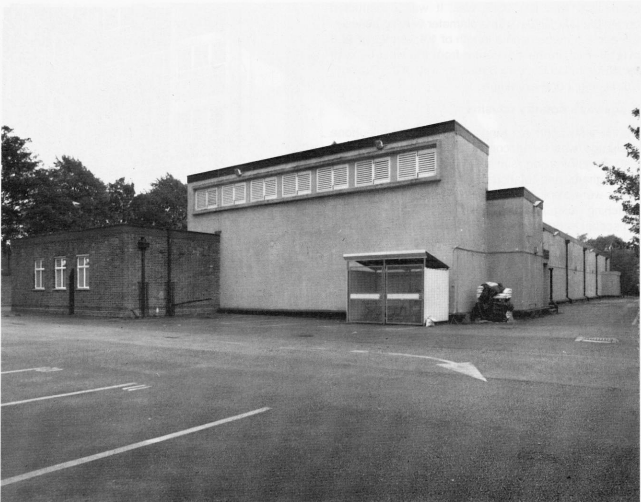
Stockport PR1 protected repeater - Photo by Nick Catford
